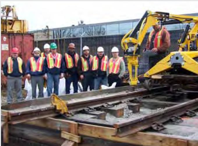
RailWorks Transit constructed a mockup of NYCT subway track at their facility in E. Farmingdale, NY, to evaluate current practices with new technology. Operations personnel observed the first test comparing a jack hammer with an electric, over-hydraulic-powered Brokk.
