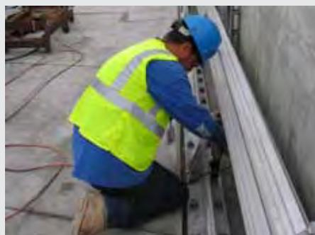
A RailWorks Track Systems employee adjusts the fixed blade portion of the switch on the APM vehicle running surface.
