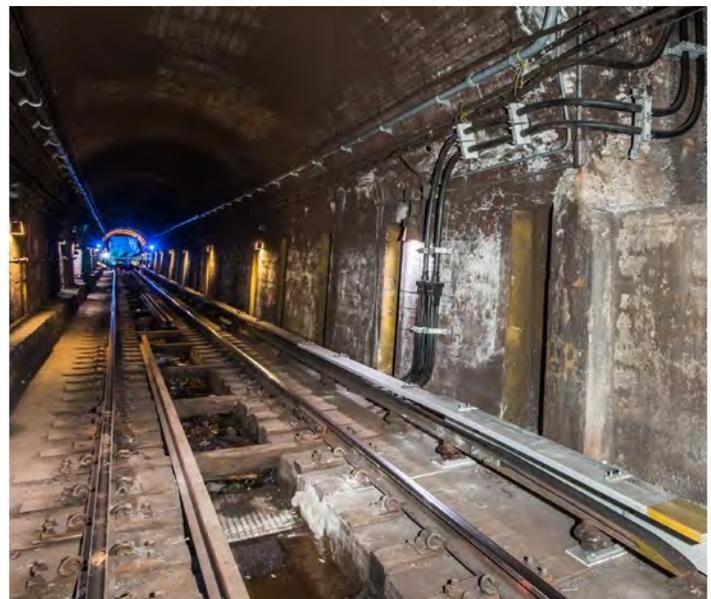
L.K. Comstock and RailWorks Transit crews worked in New York City Transit's 7 Line tunnel to install the new Vanderbilt circuit breaker house (CBH). During weekend In-Services, crews worked at track level to install new third rail and traction power cables associated with the new CBH power source.
