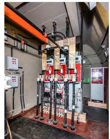
Inside the new circuit breaker house, workers installed the traction power circuit breakers and feeder cables, replacing old Westinghouse technology dating back more than 50 years.
