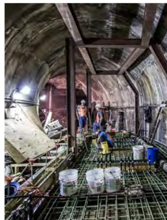
While at work in the 7 Line tunnel, workers prepared the area to pour the concrete slab within the steel structure of the new circuit breaker house.
