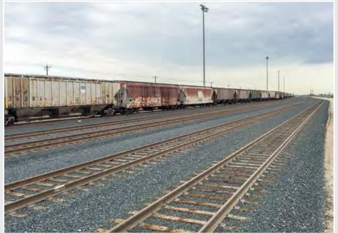
A train sits on the new 9,500-foot siding constructed by RailWorks at the Nueces River Rail Yard. In the foreground are four new ladder tracks also constructed by RailWorks at the yard, which is at the forefront of major expansion initiatives at the Port of Corpus Christi.
