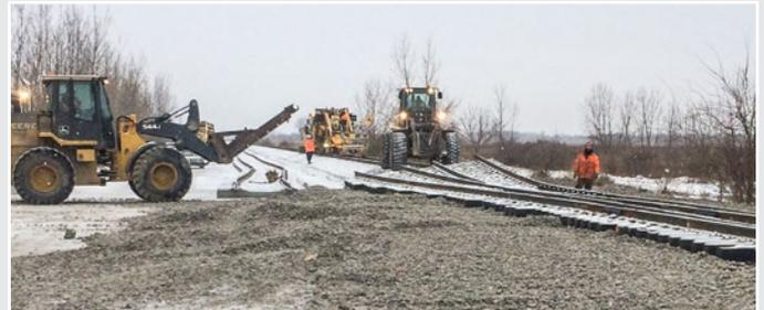
A RailWorks Track Services crew cuts a #11 turnout into a loop track leading to the BNSF Logistic Park Chicago intermodal facility outside of Chicago. Workers that day endured intermittent snow and near-zero-Fahrenheit temperatures.
