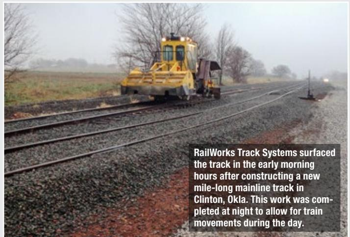
RailWorks Track Systems surfaced the track in the early morning hours after constructing a new mile-long mainline track in Clinton, Okla. This work was completed at night to allow for train movements during the day.
