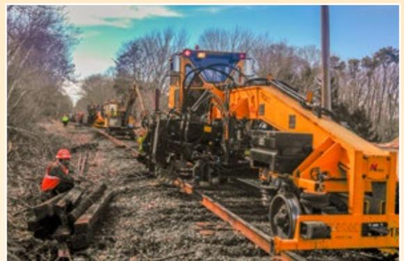
RailWorks Track Services' tie gang changed out ties on Massachusetts Coastal Railroad's Hyannis Secondary line at Barnstable, Mass., in the early spring. The crew installed more 20,000 ties over 24 miles between Buzzards Bay and Hyannis, Mass.
