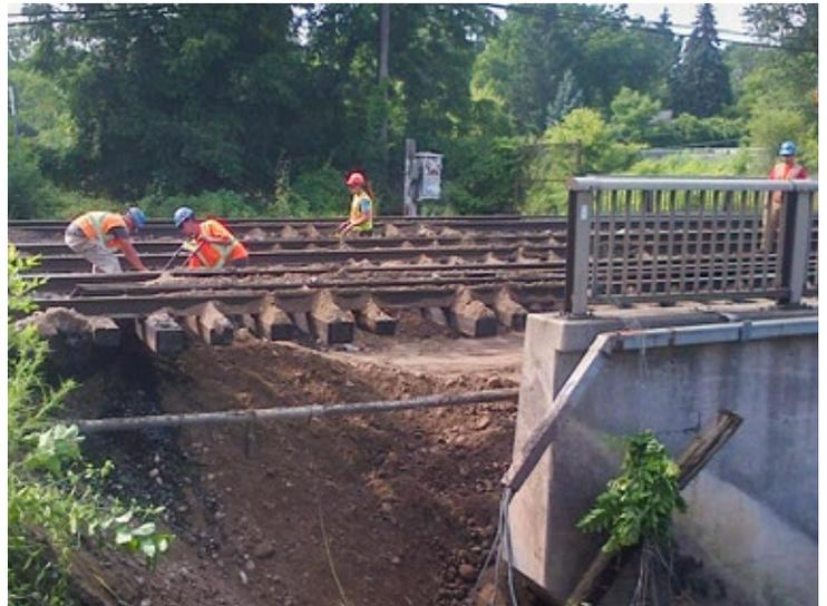
After extensive flooding caused track damage on four GO Transit subdivisions, PNR RailWorks crews worked to restore service.
