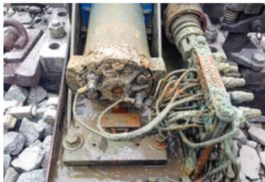
The Signals & Communications Division disassembled switch machines, saturated with mud and water, in order to clean, dry and reassemble them to make them operable.
