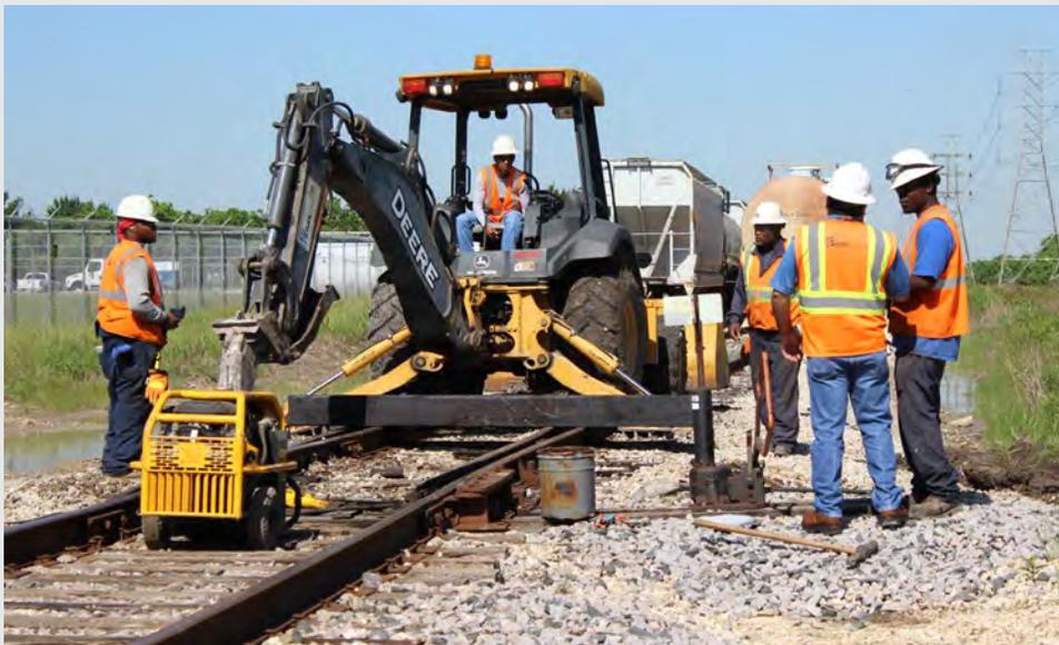
At a U.S. Development (USD) Group storage facility in Pasadena, TX, a RailWorks crew replaces a switch tie on an outbound track connecting to the UP main line. RailWorks is wrapping up a maintenance job at this plant, replacing ties and crossties on about 15 miles of track. This job is one of three RailWorks maintenance or construction projects currently under way for USD Group.
