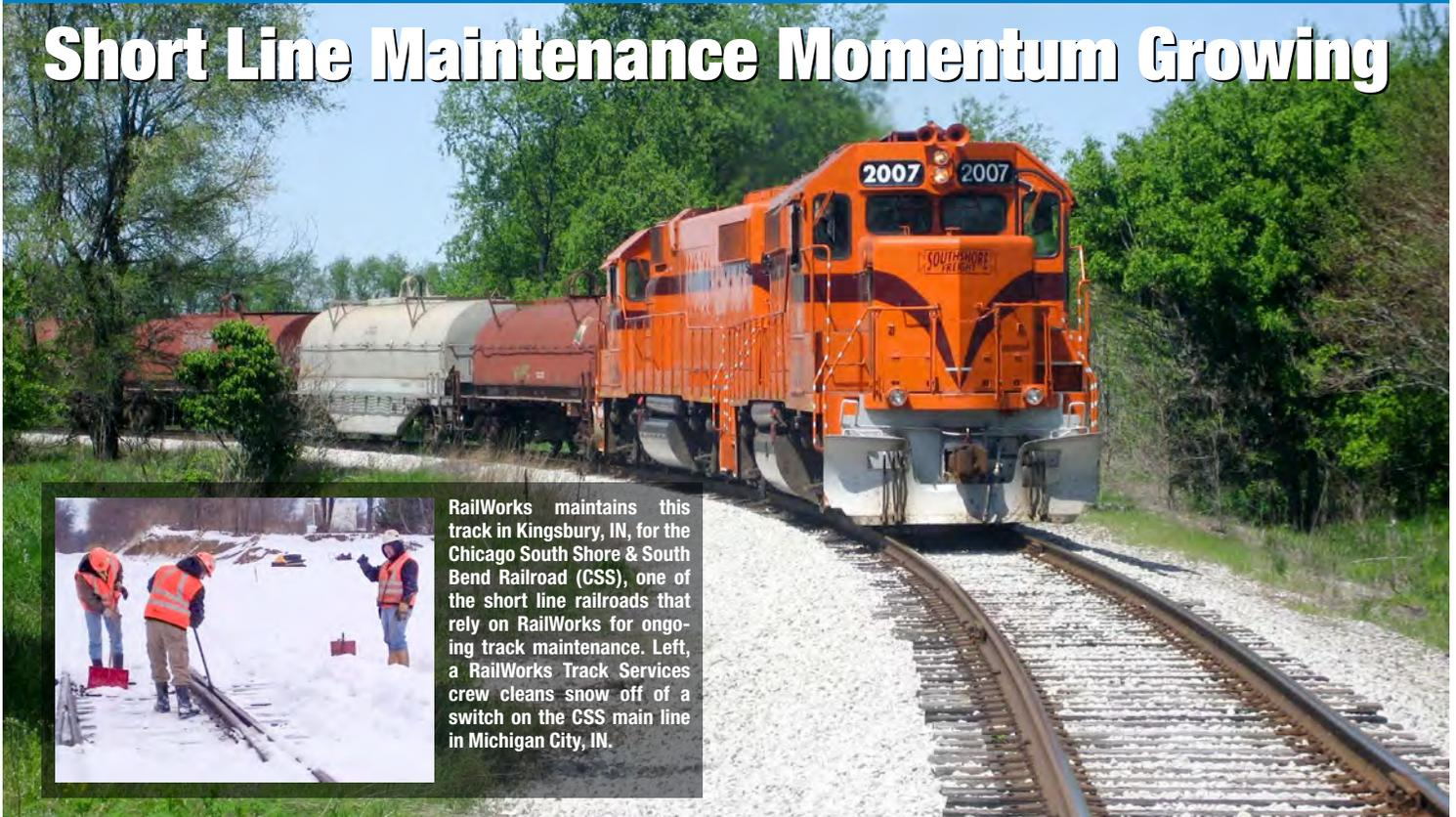
RailWorks maintains this track in Kingsbury, IN, for the Chicago South Shore & South Bend Railroad (CSS), one of the short line railroads that rely on RailWorks for ongoing track maintenance. Left, a RailWorks Track Services crew cleans snow off of a switch on the CSS main line in Michigan City, IN.
