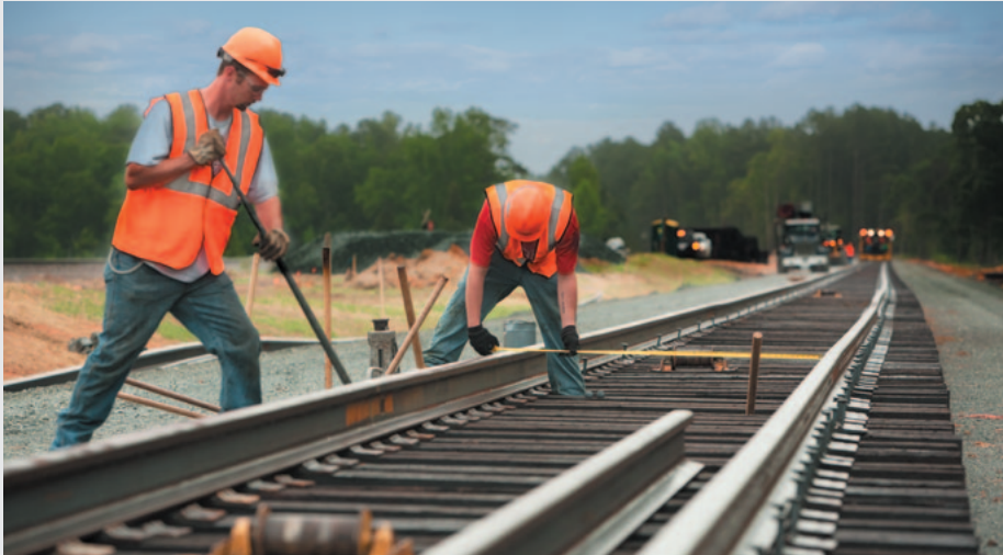
RailWorks Track Systems was not deterred from its job of constructing new track for the Western Wake Freeway project in Apex, N.C., during April, even after a tornado caused extensive damage in the area.
