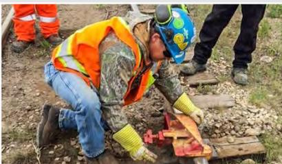
In Alberta, training focused on how to install a portable derail. Demonstrating here is Scott Redick, a trackman and operator working at Agrium's Redwater Fertilizer plant in Redwater, AB.
