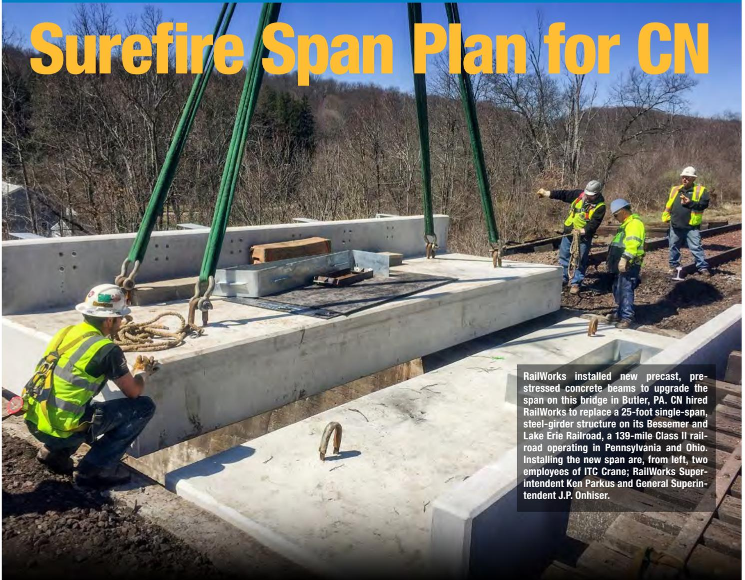
RailWorks installed new precast, prestressed concrete beams to upgrade the span on this bridge in Butler, PA. CN hired RailWorks to replace a 25-foot single-span, steel-girder structure on its Bessemer and Lake Erie Railroad, a 139-mile Class II railroad operating in Pennsylvania and Ohio. Installing the new span are, from left, two employees of ITC Crane; RailWorks Superintendent Ken Parkus and General Superintendent J.P. Onhiser.
