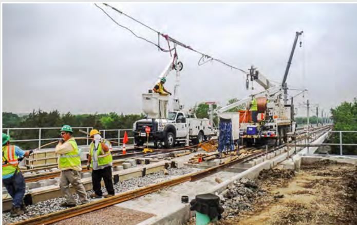
L.K. Comstock linemen pull contact wire into position for DART's new light rail extension south of Dallas, TX. Contact and messenger wires, along with the overhead catenary system (OCS) poles, work together to distribute approximately 750 volts of power to energize the light rail trains.
