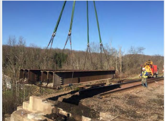
As part of the bridge span replacement, RailWorks’ Dirk Jones, laborer, assists in the removal of steel girders, making way for RailWorks to install a precast, prestressed concrete, ballast-deck span.
