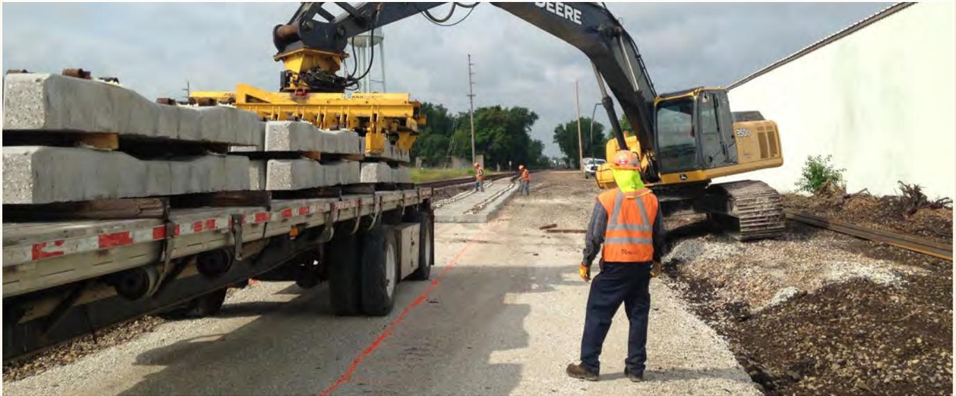
RailWorks Track Services employees in Lincoln, IL, bed concrete ties to be used to construct a new siding there as well as a #11 turnout.
