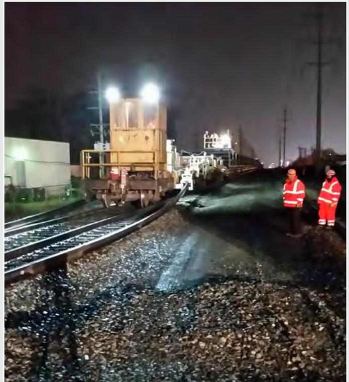
L.B. Foster employees are ready to help a RailWorks crew unload quarter-mile-long strings of continuous-welded rail (CWR) from this work train. Because CWR features fewer joints, it helps provide the necessary rail strength for handling trains at higher speeds and creates a smoother ride for passengers.
