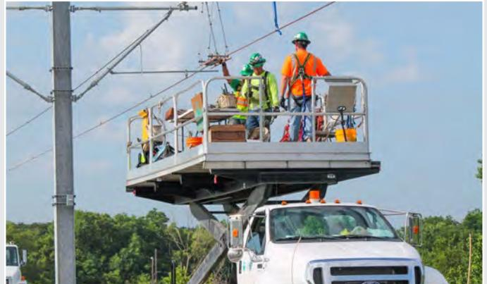
During a cutover in July, L.K. Comstock workers completed the interface of the newly installed overhead catenary system on the Dallas Area Rapid Transit agency's new Blue Line extension with the existing Blue Line.
