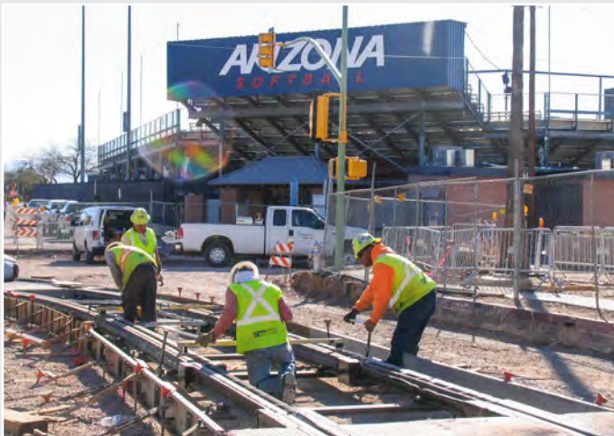
In March, RailWorks Track Systems employees at work on the streetcar route check pre-curved track at East 2nd Street on the University of Arizona campus.
