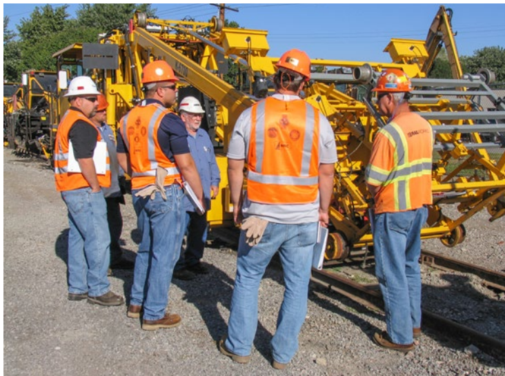
RailWorks employees discuss machine safety with Progress Rail shop employees before examining a Pandroll Jackson K6700 tamper.
