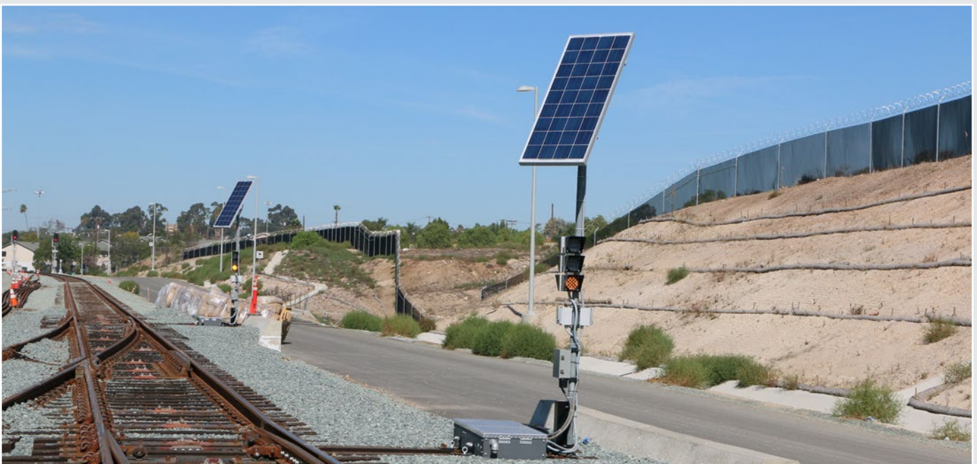
RailWorks completed a range of track improvements at the San Ysidro Freight Yard, including the installation of these two solar-powered GE switch machines.
