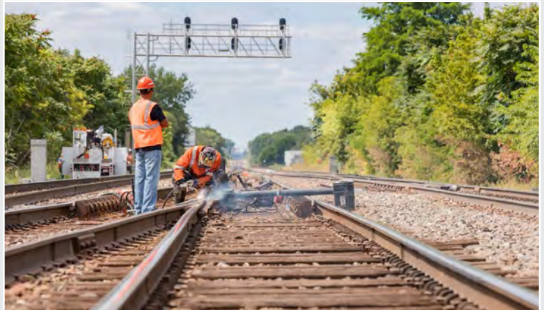
Helper Eric Balsler performs electric welding to repair a frog on BNSF Railway's main line in Naperville, IL, while Welding Supervisor Kris Hyder looks on and provides additional lookout protection for train traffic on adjacent tracks.
