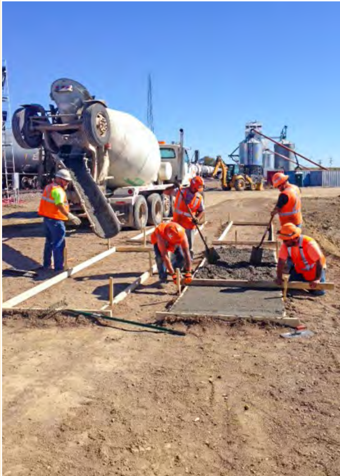
At left, employees working near Pillsbury, ND, have built forms and are finishing the concrete pads for four large propane tanks that will fuel heaters for a switch on BNSF Railway track. A cement truck driver watches RailWorks' Crewman Craig Knowles (front left) and Foreman Derrick Stratton. Behind them are Crewmen Anthony Akel (left) and Brandon Hawkings. In the photo at right, that same crew used a tag line to position a ground wayside signal onto its foundation, after which they finished the installation by bolting the signal to the foundation. Tom Johnson is operating an all-terrain lift.
