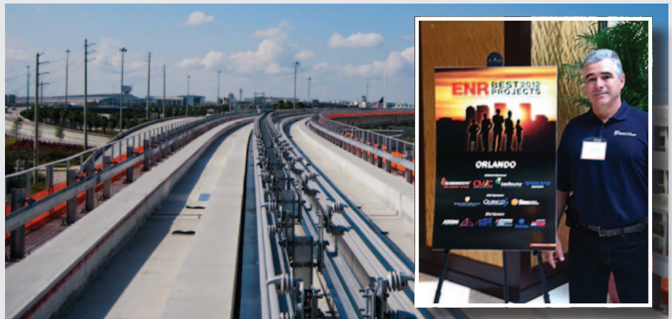
Quality Control Manager Tomas Ramos represented RailWorks Track Systems at the ENR Southeast "Best Projects" awards ceremony in Orlando on November 15. The MIA Automated People Mover project was recognized as a "Best Project" as well as for overall safety. In early 2011, RailWorks completed work on this project to install the guidance system, power rail, six switches and a wash platform for APM vehicles at Miami International Airport.
