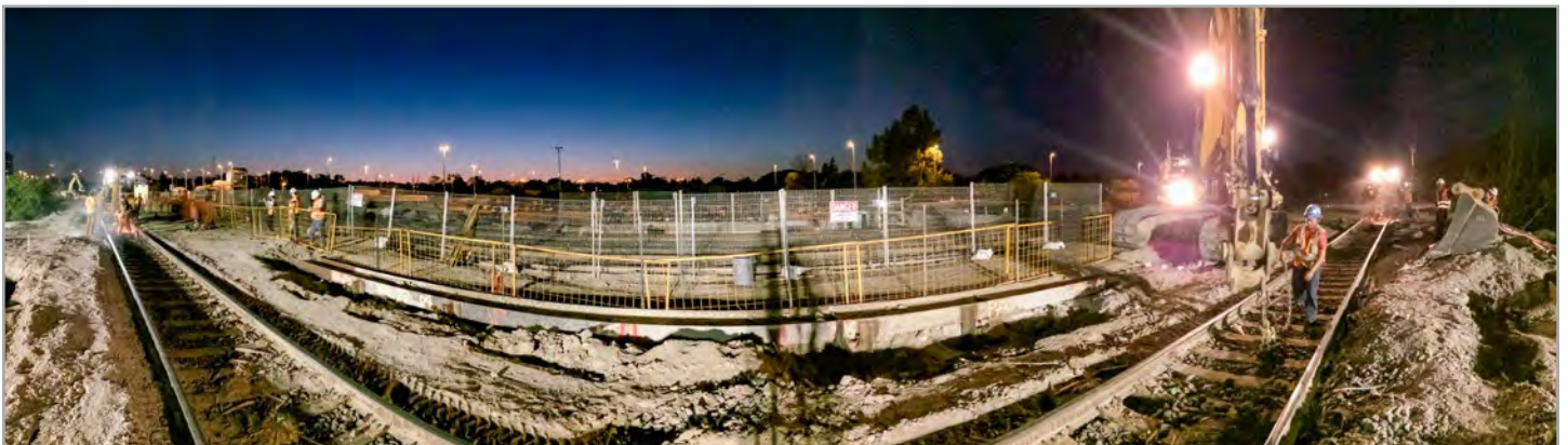
During a 53-hour weekend outage, PNR RailWorks track, signals & communications and GO Transit Maintenance crews helped with the installation of pedestrian tunnels near the GO Transit Guildwood Station west of Toronto.
